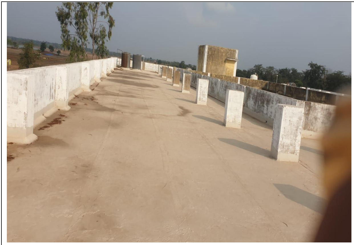
Proposed Site for 10kwp Solar Power Plant
